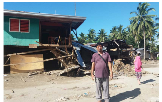
Credit: OCHA/R. Maquilan Salvador, Lanao del Norte (30 December 2017) - Kusain Ibra stands in front of his home, which was destroyed by floodwaters during Severe Tropical Storm Tembin.
