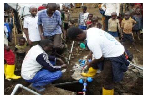
REHABILITATION OF A WATER SUPPLY NETWORK, NORTH-KIVU. © IOM MAY 2017 (C. FRISONE)
