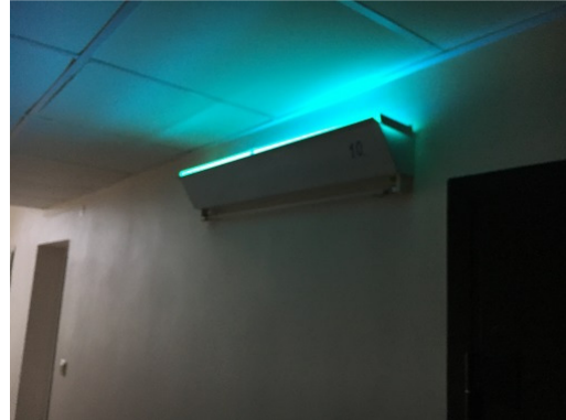
Fig. 4b. Shielded ultraviolet germicidal irradiation fixture
