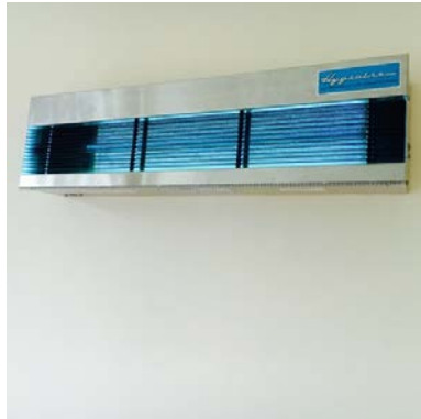
Fig. 4a. Louvered ultraviolet germicidal irradiation fixture
