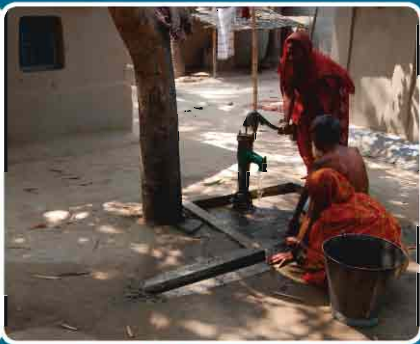
Surrounding of the tubewell is clean and no water stagnates there. The drain is clean and the used water drains out
