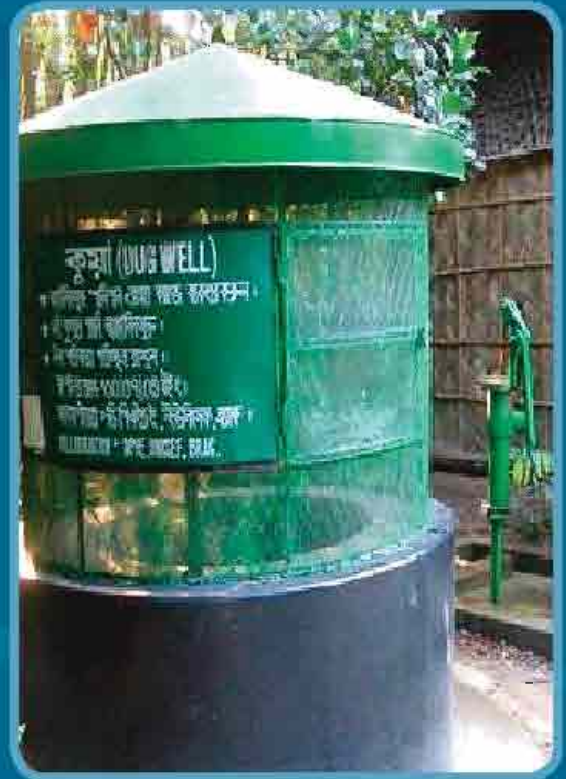
Ring Well / Dug Well
