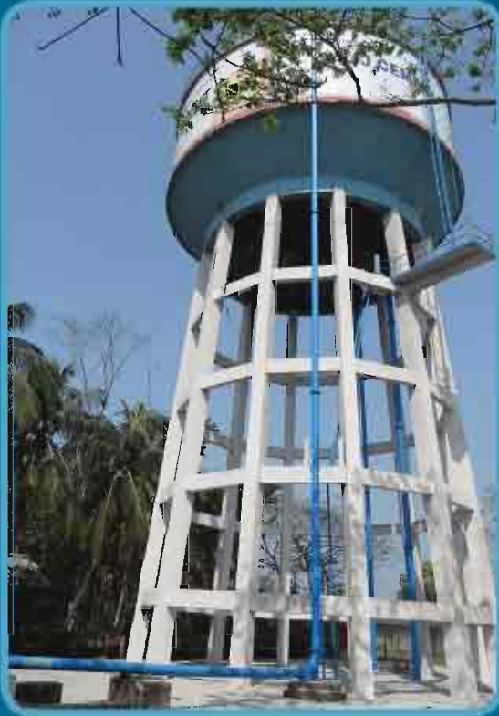
Piped water supply system
