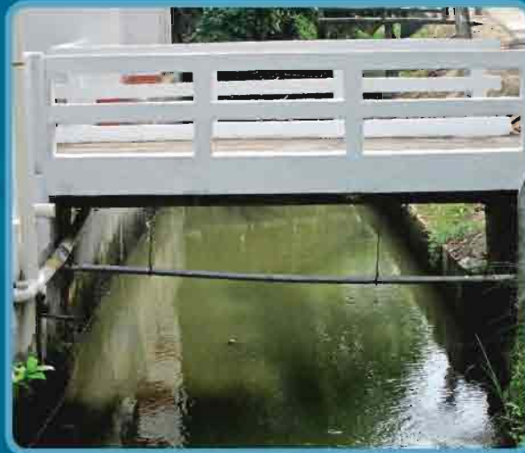
Connections are proper and supported in pipe crossing over canal/drain
