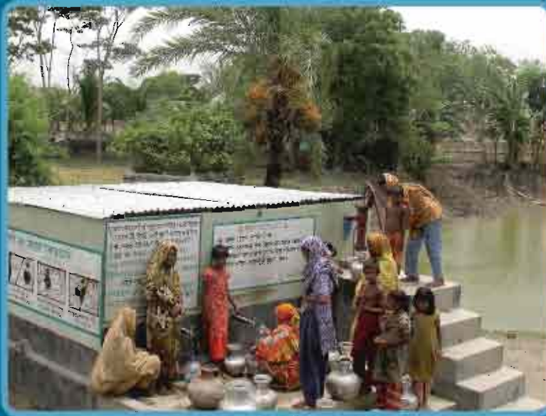
Pond-Sand Filter (PSF)
