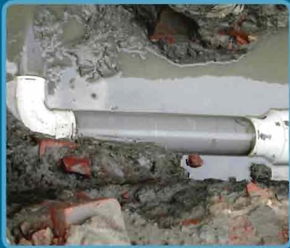
Connections are made properly in pipe
