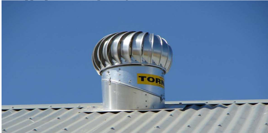
Figure 4: Example of roof mounted turbine ventilation, or “whirlybird”, highly appropriate for improving ventilation in warm climates.
