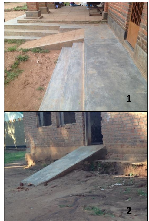
Figure 2: ramps at resource centre (1) and mainstream (2) schools
