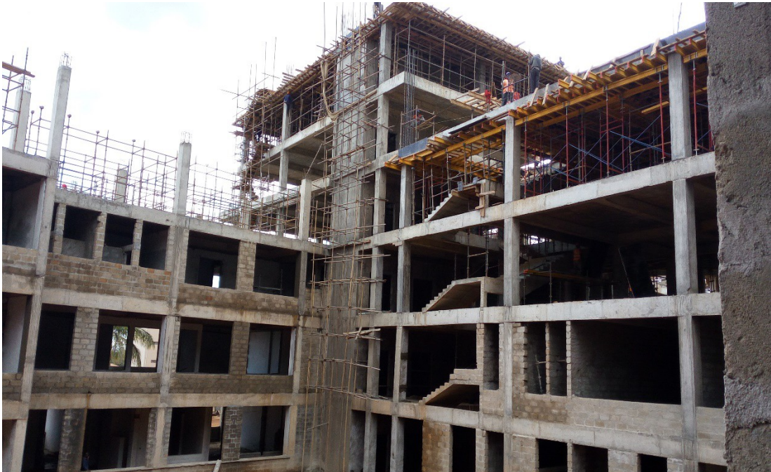
Works continue to be undertaken at levels 4, 5 & 6
