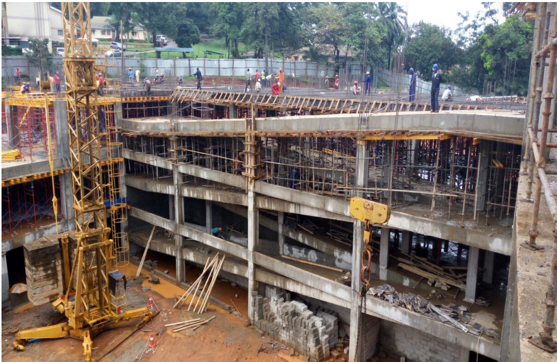
Construction of the connecting ramp in progress
