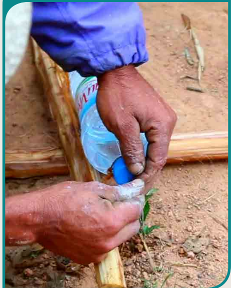
Constructing a handwashing station
