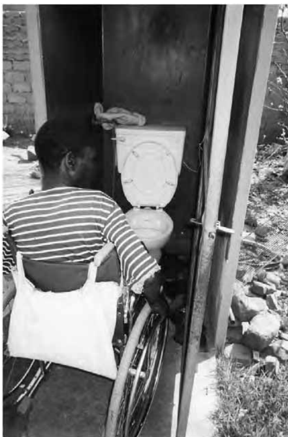
Figure 23.2: Inaccessible toilets in RDP houses
