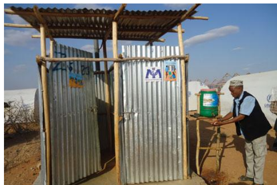
Figure 6: Latrine construction in a refugee camp (IMC)
