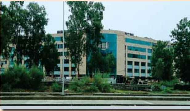
Newly constructed AIIMS Rishikesh
