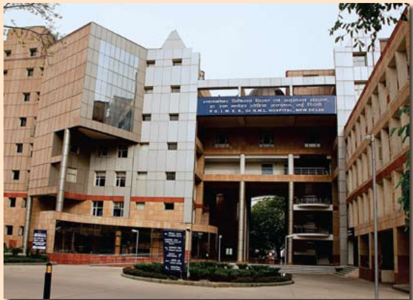
Newly constructed emergency block of Dr. R.M.L. Hospital, New Delhi
