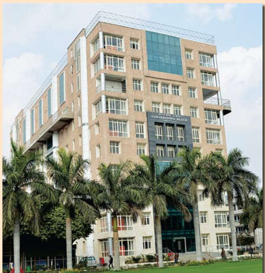
Newly constructed Convergence Block, AllMS 2013-14
