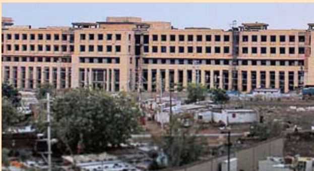
Newly constructed AIIMS Bhopal
