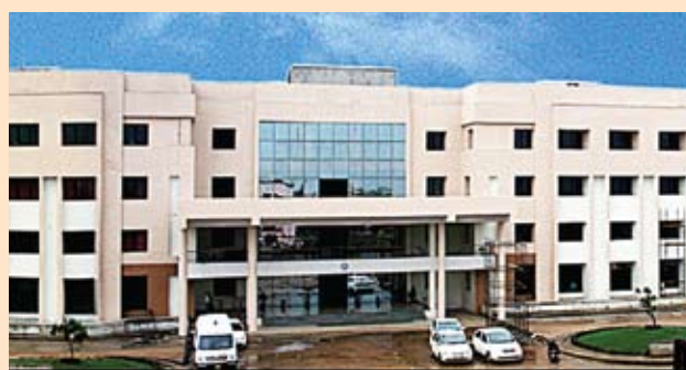
Newly constructed AIIMS Raipur
