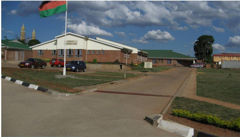
Bwaila Maternity Hospital, Lilongwe
