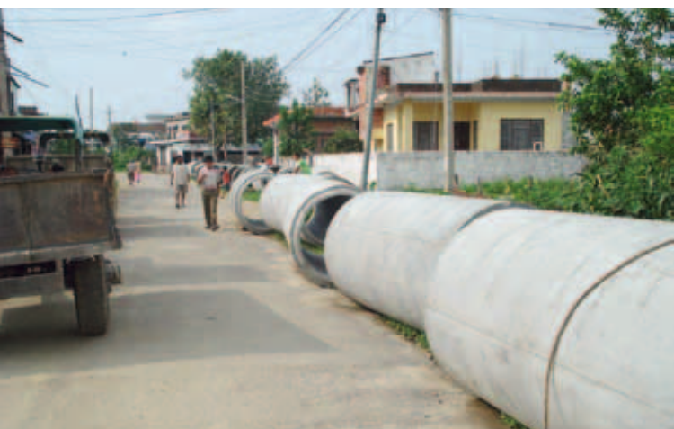
Photo7j: UEIP project in Hetauda installing new drains © UN-HABITAT
