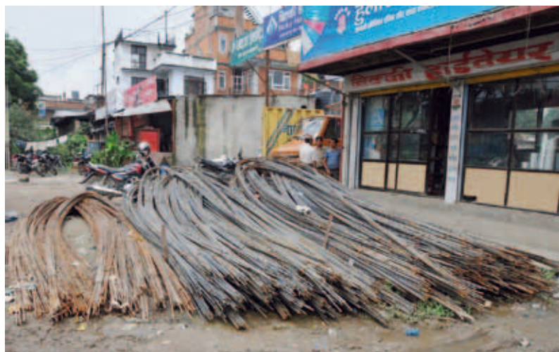
Photo8d: Reinforcing steel rods for Pakki housing © UN-HABITAT
