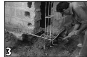
3 Chisel the existing plinth beam/band without destroying the existing reinforcement
