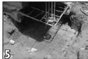
5 Clean the surface of the P.C.C. and place #3 bars @ 8" spacing on both ways in the form of mesh over P.C.C. surface
