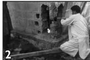
2 Remove the masonry in tooting pattern
