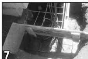
7 Place shuttering for plinth for pouring concrete
