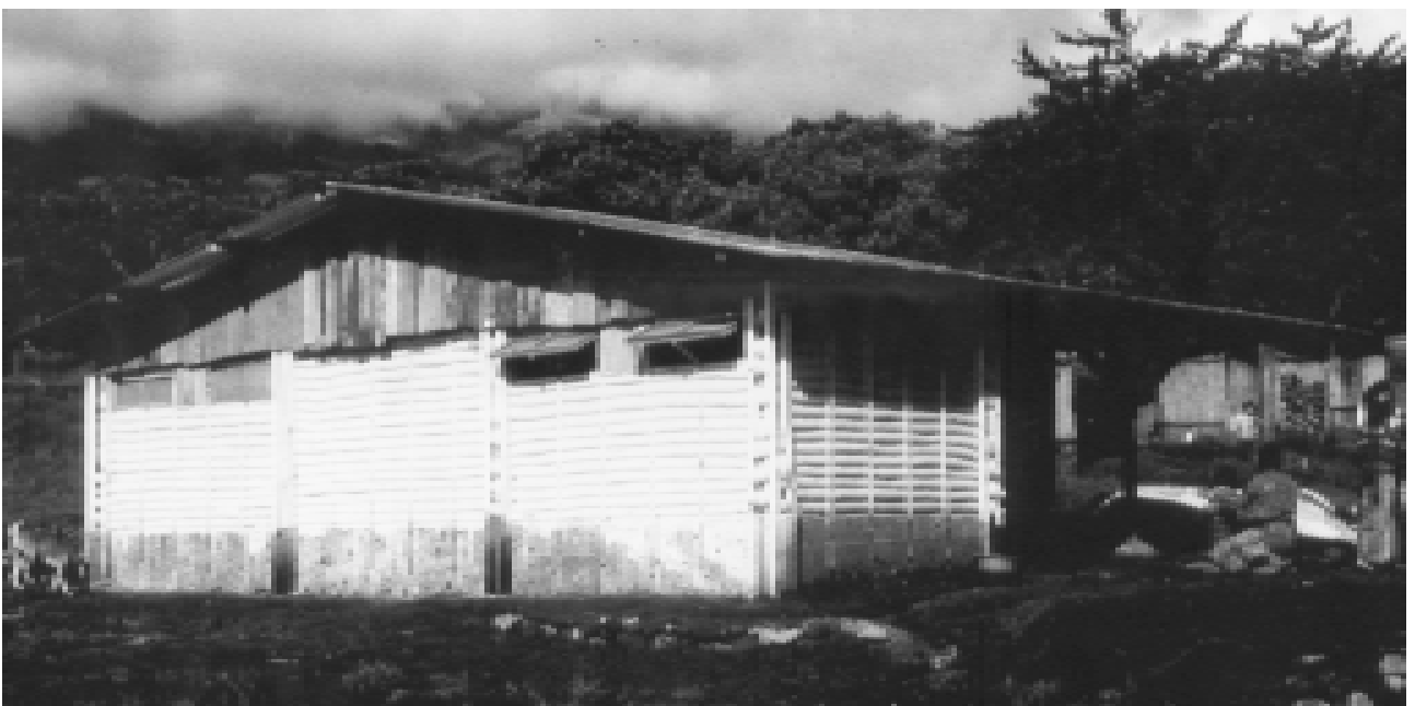
9-7 Earthquake resistant low-cost housing prototype, Guatemala 1978
