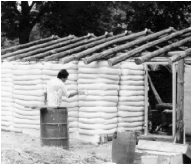
9-2 and 9-3 Wall with filled textile hoses
