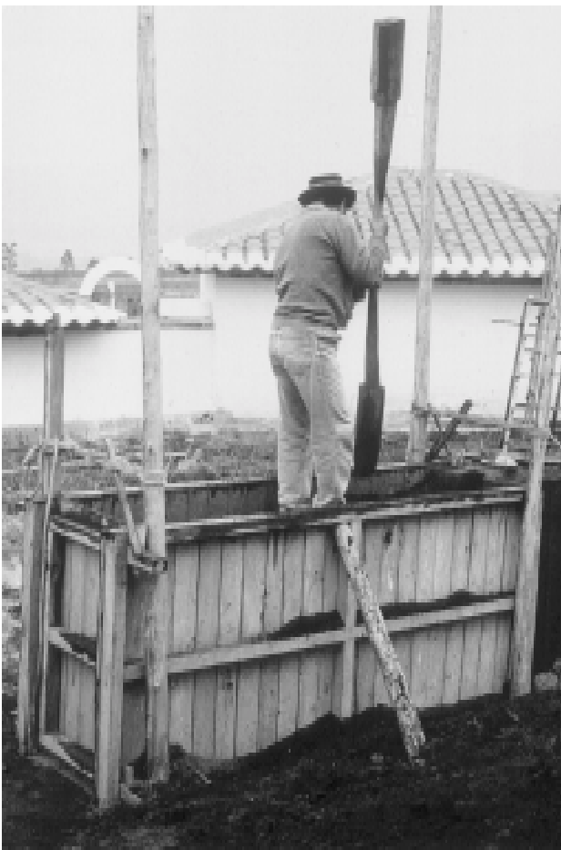
6-2 Temper with two «heads», used in Ecuador (Minke 2001)
