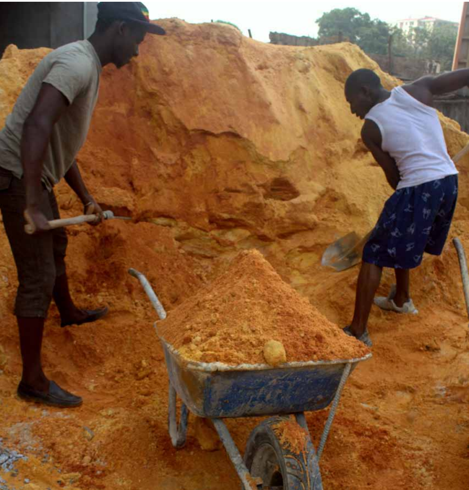
Construction work in Conakry, Guinea. (Photo: Anne Kennedy/UNDP)
