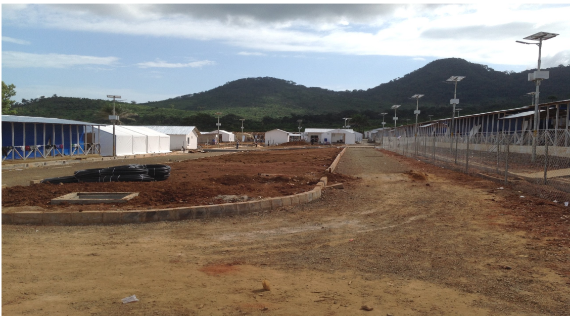
Kerry Town Treatment Centre During Construction
