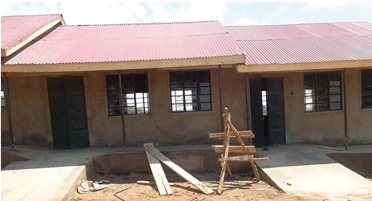
Image showing classrooms constructed at Nangina Special School
