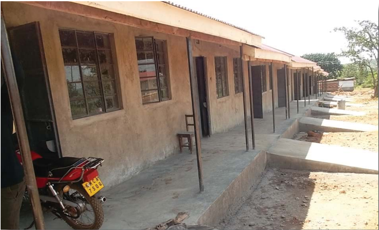
Image showing classrooms constructed at Nangina Special School
