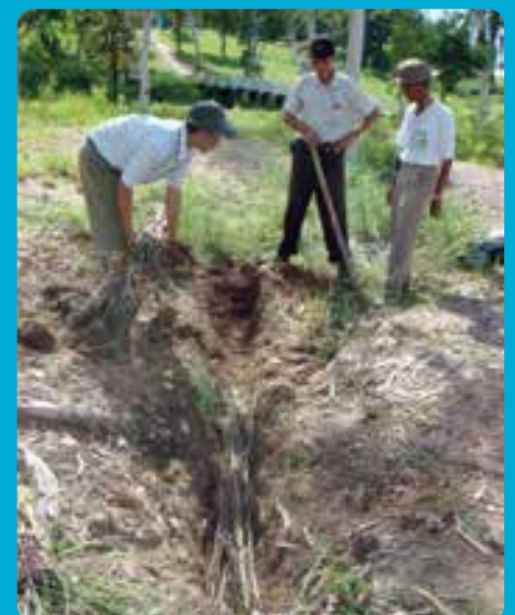
Figure 18: Installing live fascine
