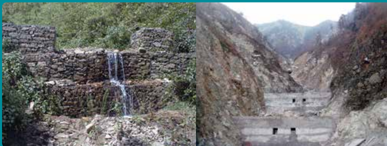
Figure 37: Gabion check dam (left) and masonry check dam (right)
