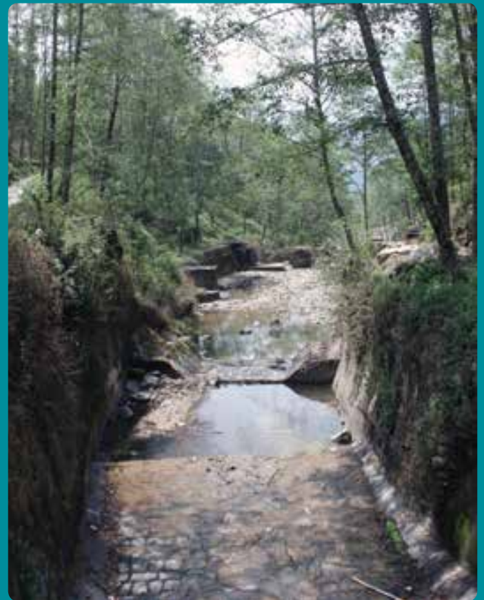
Figure 67: Concrete channel lining
