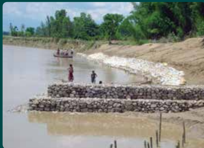
Figure 42: Gabion spurs with sandbags along the bank
