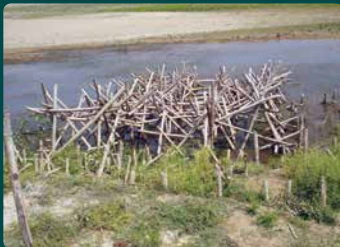
Figure 50: Bamboo porcupines used to form a spur
