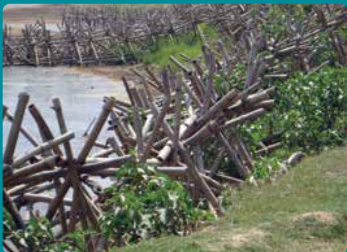
Figure 63: Bamboo porcupines as protection along an embankment
