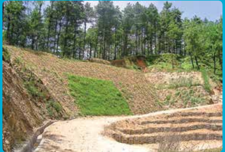
Figure 6: Bioengineering for soil conservation
