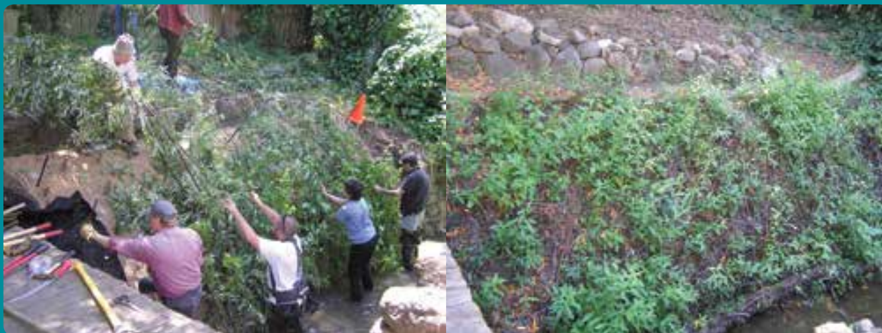
Figure 12: Installing brush mattress
