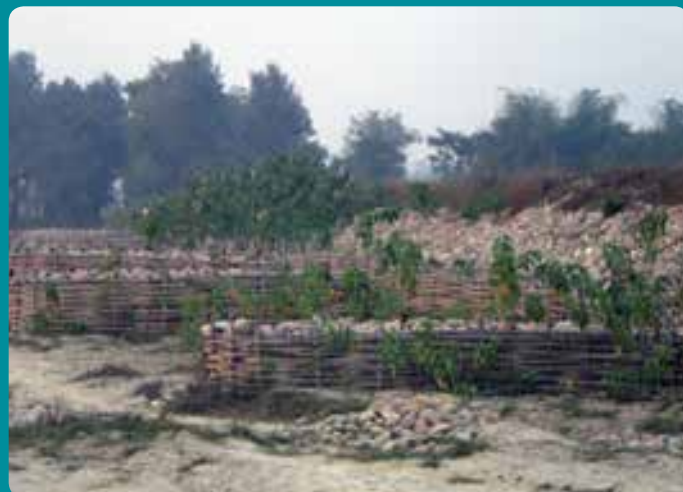
Figure 43: Low-cost bamboo and stone spurs
