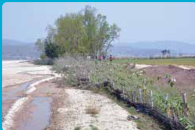
Figure 21: Wattle fence used for river bank protection
