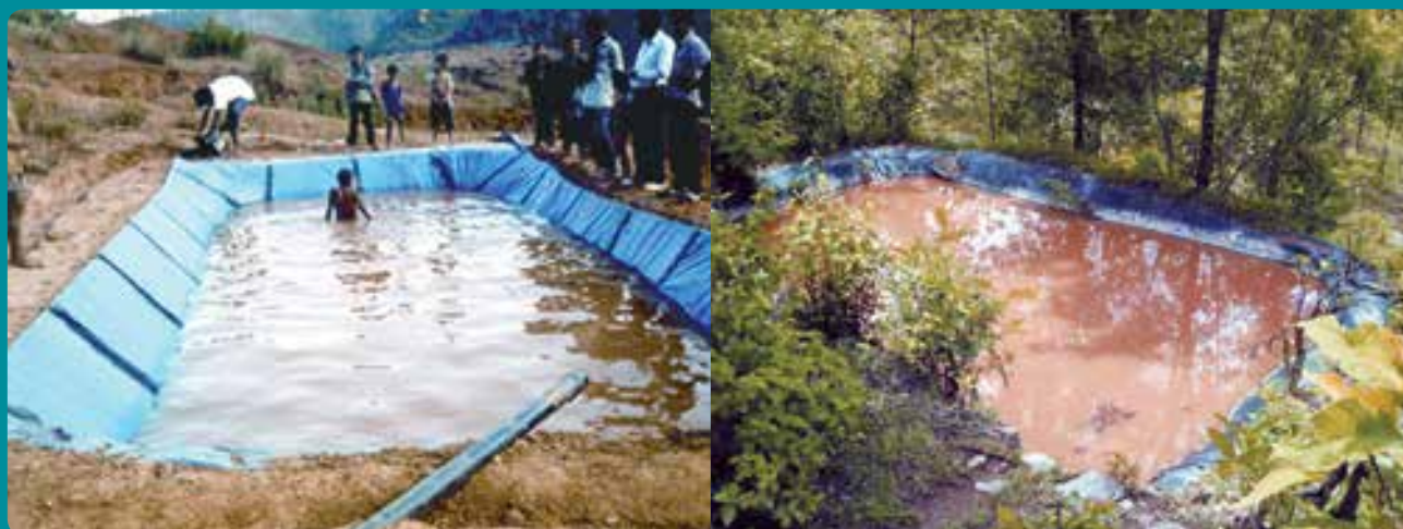
Figure 31: Earthen ponds laminated with plastic sheet
