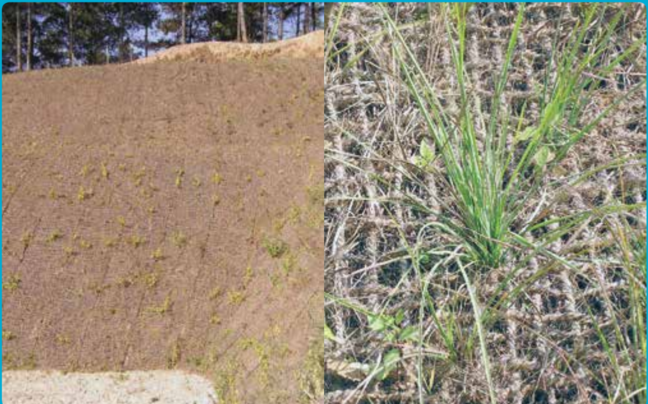
Figure 15: Jute netting on a cut slope
