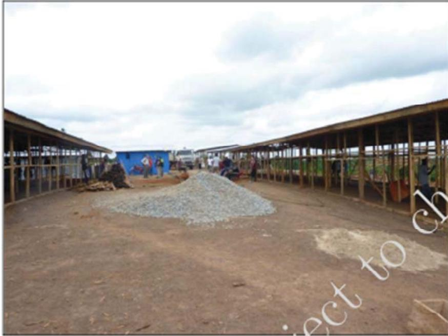
Use of gravel to prepare the ground for ETU construction on earth-exposed areas
