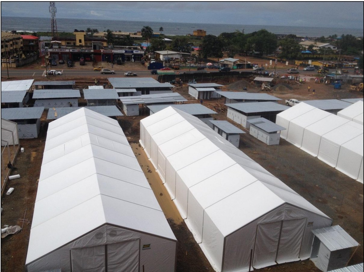
Ministry of Defence site, Congo-town, Monrovia, LIBERIA
