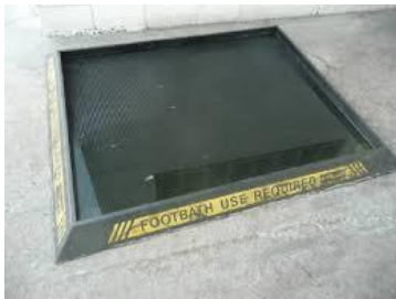
Chlorine foot bath
