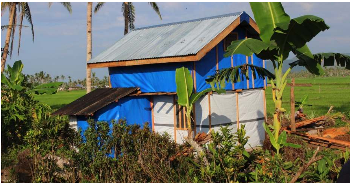
A shelter kit with temporary tarp walls
