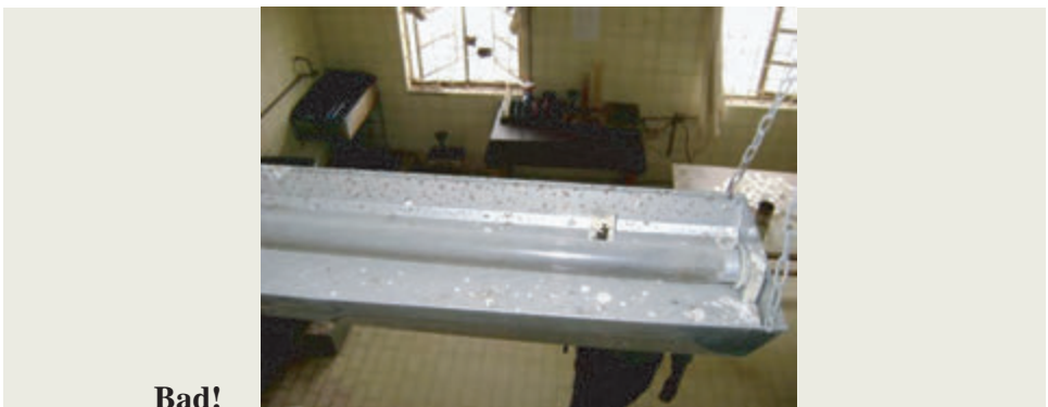
Non-functioning, not cleaned UVGI fixture
