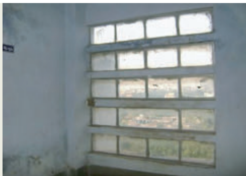
Windows sealed with renovation
