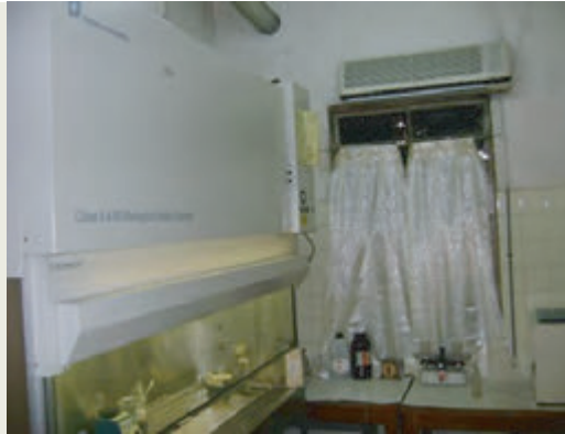
Air conditioner in front of Biosafety cabinet
