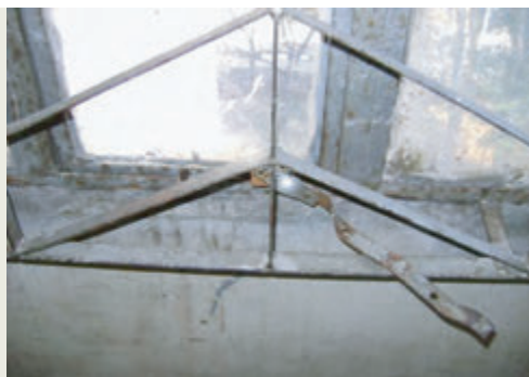
No maintenance of moving parts of window
