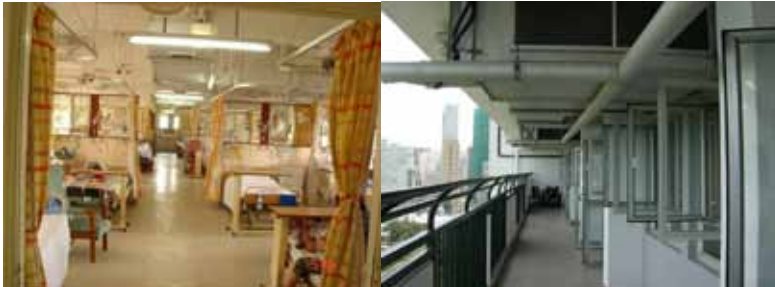
Figure G.1 Open wards and windows in the tuberculosis ward in Grantham Hospital
