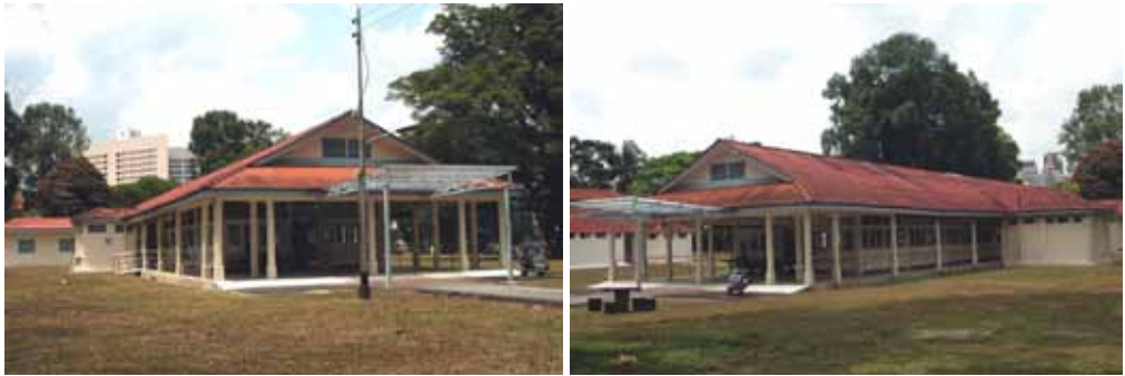
Figure H.1 Two views of the single-storey tuberculosis inpatient ward; the perimeters are free from obstruction, allowing natural ventilation throughout the year
