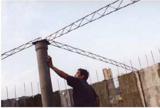
Figure 15. Fixing of Roof Trusses (Stiffeners)
