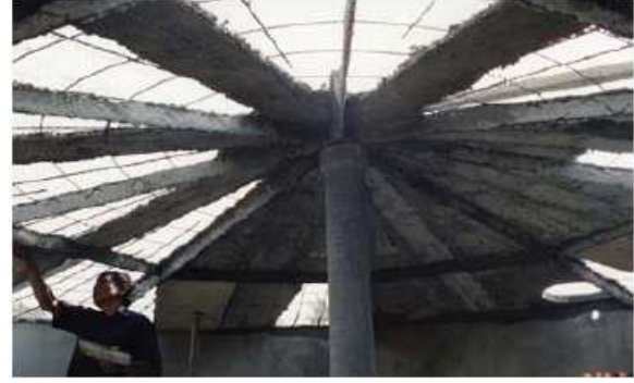
Figure 19. Plastering of Roof
