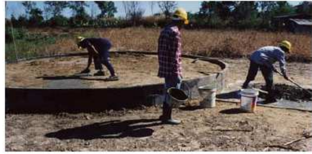
Figure 5. Preparation of Lean Concrete Base
