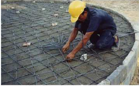
Figure 6. Placement of Rebar for Base Slab
