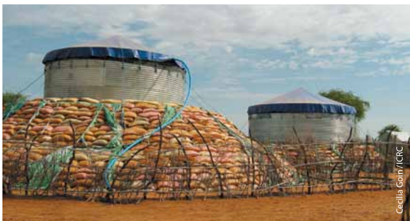
Figure 18 Emergency water storage facilities
