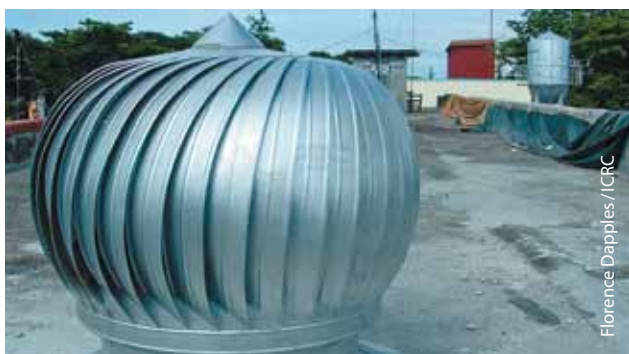
Figure 16 Natural ventilation system not using electricity (when possible)
