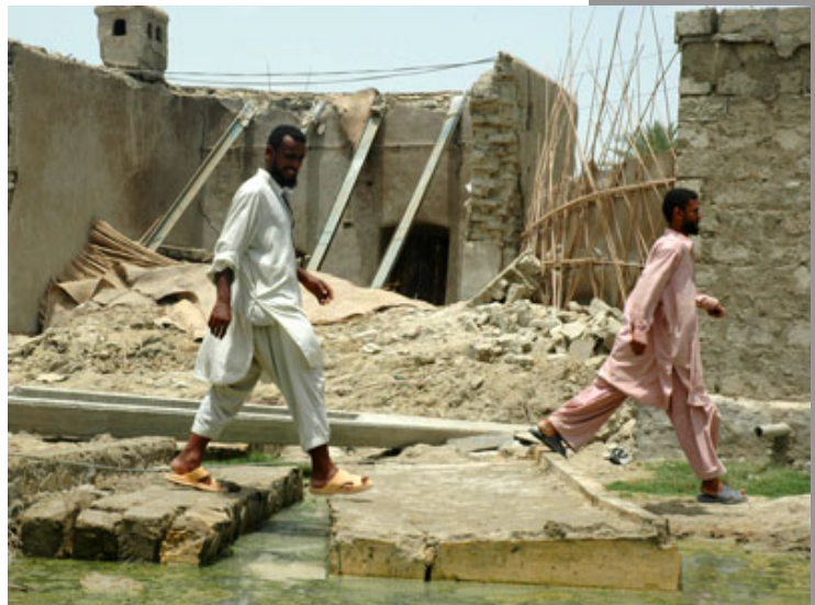
Two men walk along a broken concrete sanitation drain in Nokalat, Pakistan. Photo: Mubashir Fida/ International Federation
