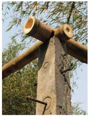
Step 2.D: top plates lapped and bolted at corners
