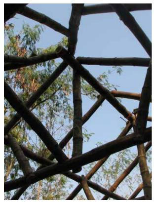
Step 2.G: diagonal braces from bukpar to tie-beams
