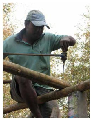
Step 2.E: tie beams pre-drilled and nailed
