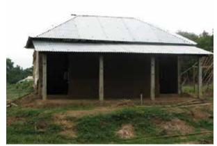
Step 4.C: ridge covers attached to CGI sheetsroof structure at ridge and diagonals
