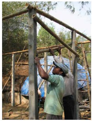
Step 2.D: cross-braces bolted at corner pillars
