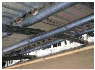
Step 4B: CGI sheets attached to tertiary roof structure with U-hooks, rubber and diamond washers
