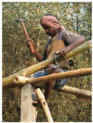
Step 2.E: diagonal primary roof supports pre-drilled and nailed
