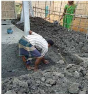
Step 3.A: plinth constructed and compacted to floor level
