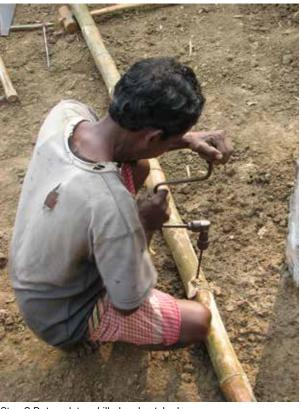
Step 2.D: top plates drilled and notched
