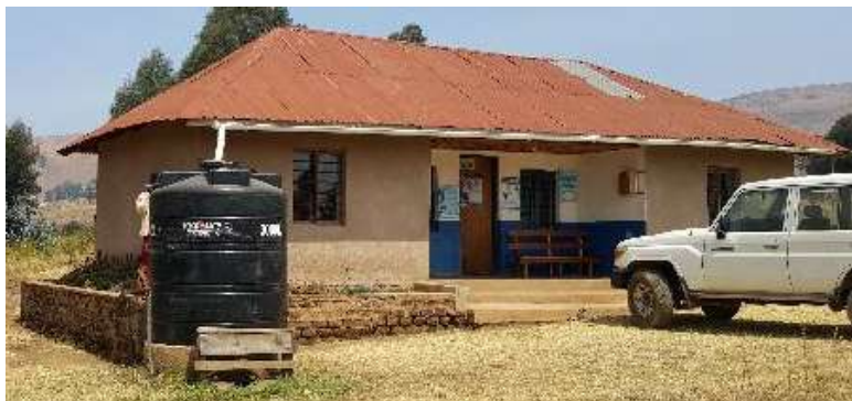
Figure 11: Rain water harvesting and storage tank at a dispensary. Rain water harvesting system was provided supplementary to intermittent piped water supplied at a standpipe.
