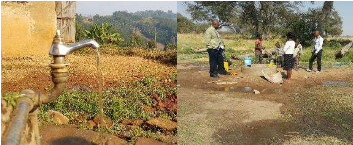
Figure 5: Water sources as observed in some HCFs, a stand pipe outside of a facility with plumbing (left) and an open but lined well used by another facility (right).
