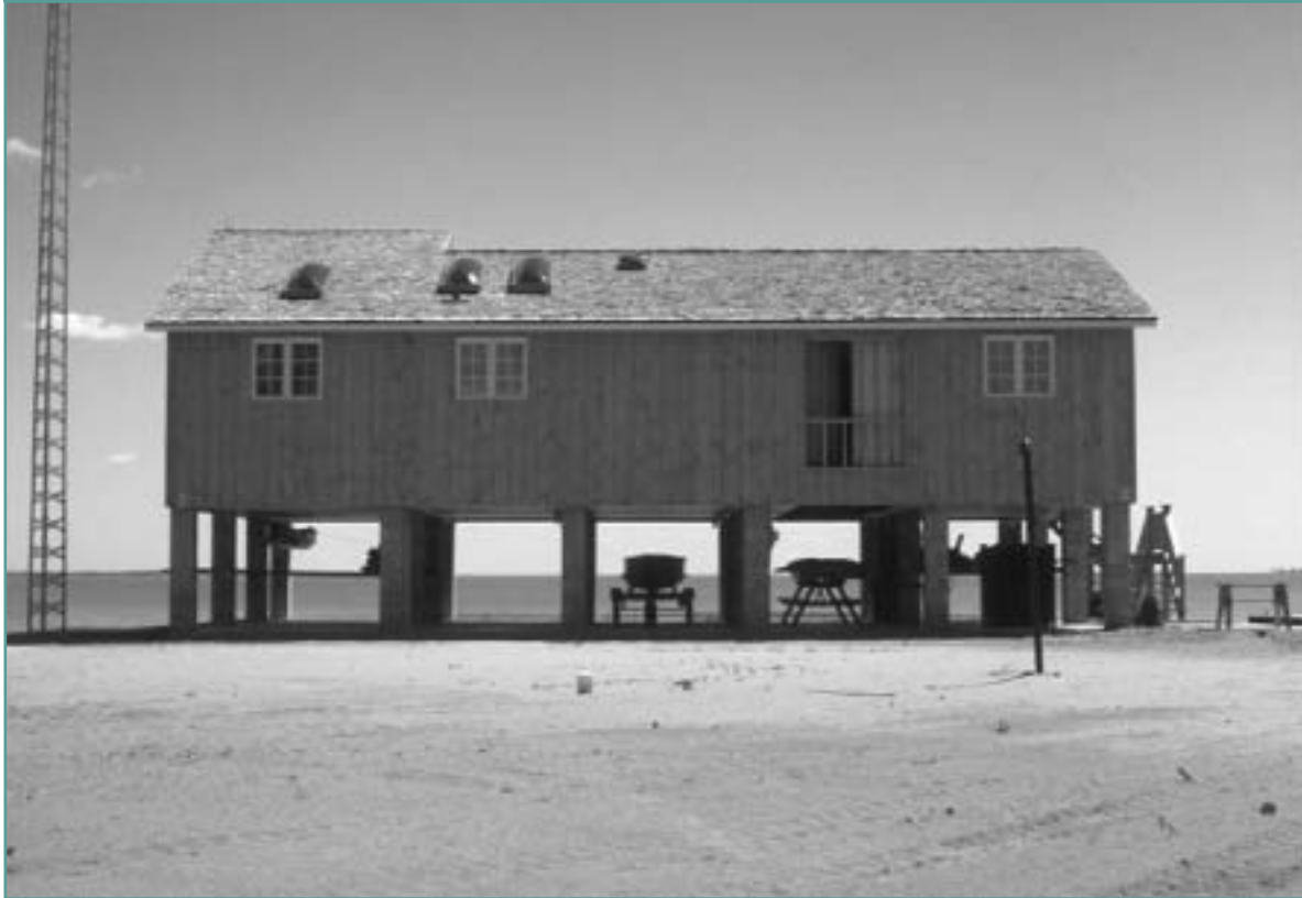
Flood proofed dwelling
