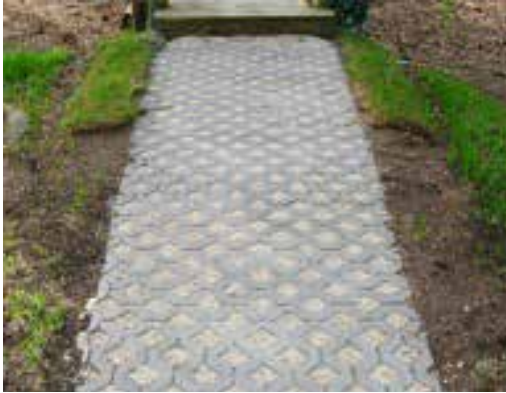
Installed permeable pavers 17
